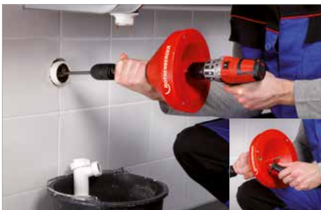
Electrical operation with cordless drill
